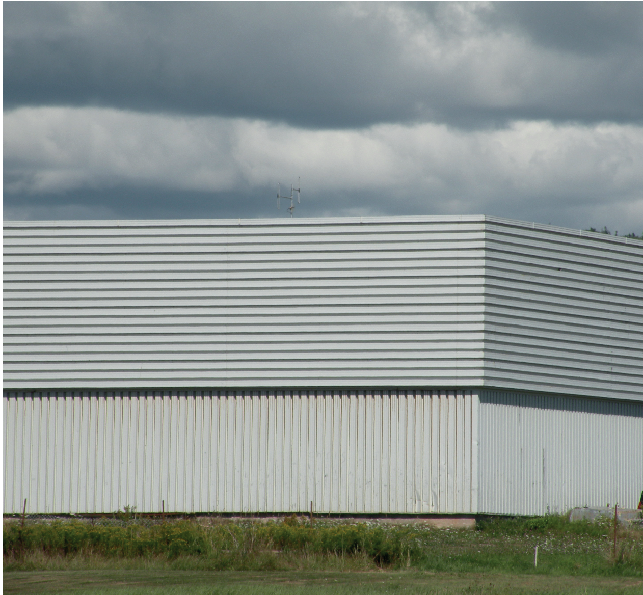
Tom McGlynn. metal pre-fab building, Judique, Nova Scotia, August 2013.
